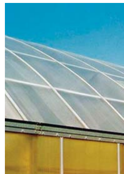
Image shows greenhouse glazed with DEGLAS acrylic roofing and polycarbonate walls. Both the acrylic and the polycarbonate glazing are of similar age. This image has not been altered in any way.
