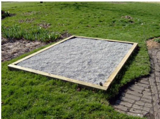
The length of these anchors should be no less than 12" depending upon the type of soil (loose or compacted) in your area. Now that you have finished building a foundation for your new greenhouse, the inside should be filled with 2 to 3 inches of pea gravel (see right), wood chips or some type of material that will allow for good drainage. Obviously, this task is much easier if it is done before securing the greenhouse
